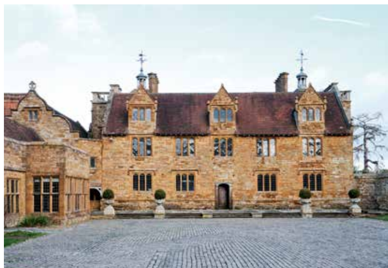
ABOVE The original entrance facade of Ashby Manor House with its mullioned windows and handsome gables.
